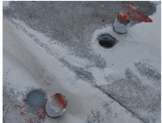
Figure 7. Core drilling
