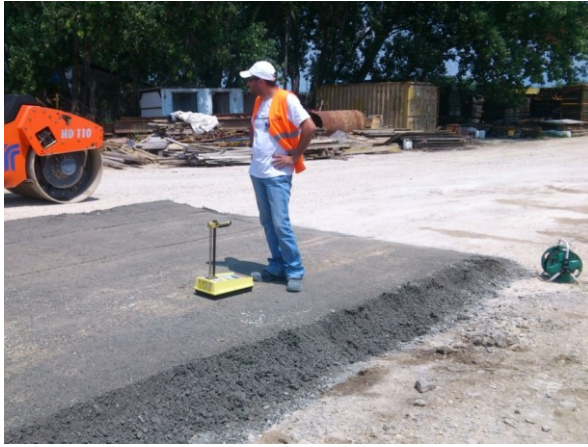
Figure 4. Fresh concrete density measured with nuclear gauge
