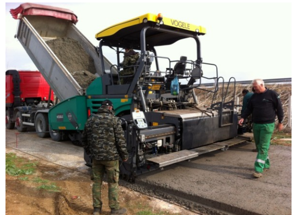
Figure 2. Truck unloading onto paver and RCC laying
