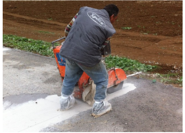
Figure 6. Joint cutting
