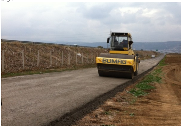
Figure 5. Roller compaction of pavement
