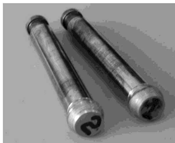
Fig. 7.14. Corrosion of rods made of steel 25H1MF in the zone of contact with gland stuffing:
