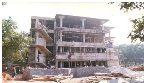
Fig. 4. storey building constructed using flyash bricks at Indian Institute of Technology, New Delhi
