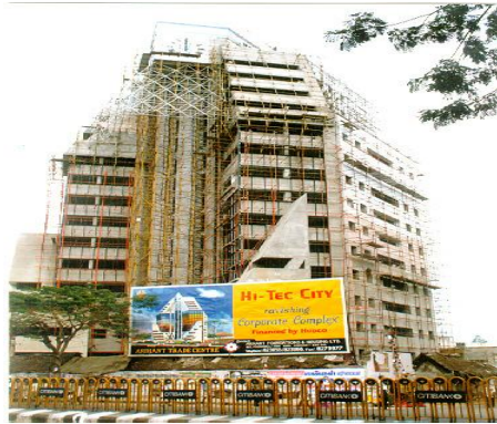
Fig.8. Use of fly ash based cellular light weight concrete at Chennai
