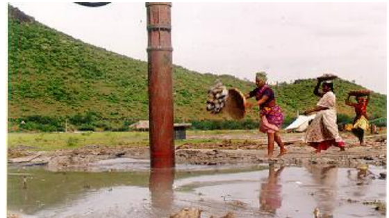
Fig.11. Densification by Vibroflotation, Vijaywada Thermal Power Station, Andhra Pradesh
