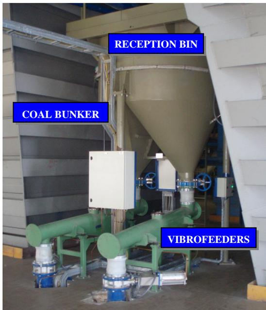
Fig. 3. Reception bin located between the coal bunkers
