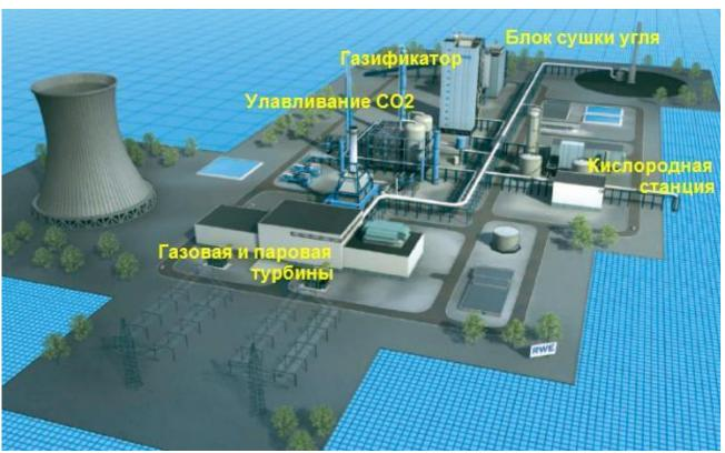
Capacity of the unit -450 MW (net capacity of 330 MW). Efficiency factor -35%, including transport and burial of  $CO_2$ . Volume of  $CO_2 - 2.6$  million tons a year. Capital expenses -1.7 billion € (2007), including transport and burial of  $CO_2$ .
