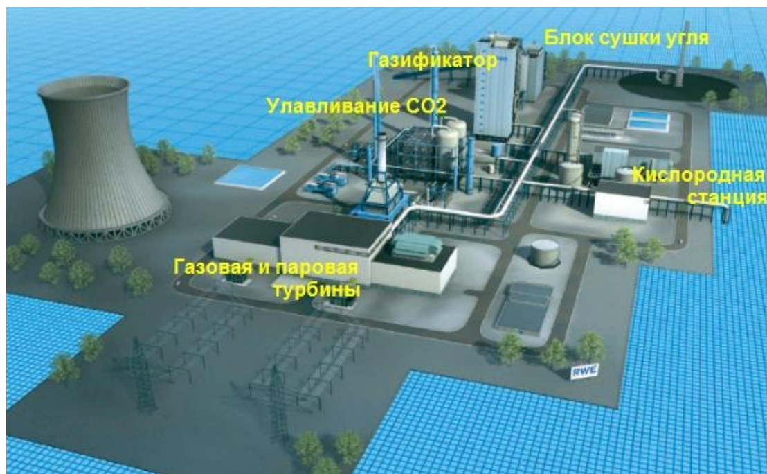
Fig. RWE project: combined cycle GT with brown coal gasification and O 2 capture (2014): блок сушки угля - coal drying unit, кислородная станция - oxygen station, газификатор - gasifier, улавливание CO 2 - CO 2 capture, газовая и паровая турбины - gas and steam turbines. Capacity of 450 MW (330 MW net); efficiency of 35 %, incl. CO 2 transportation and storage. Amount of CO 2 captured makes 2.6 mln tCO 2 /year. Capital cost - €1,7 bln (2007), incl. CO 2 transportation and storage.
