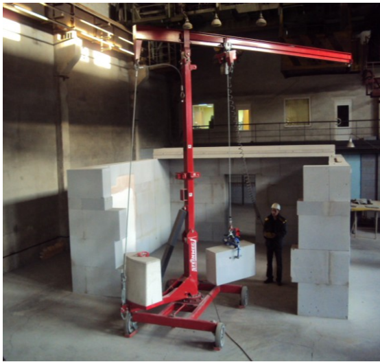
Fig. 3. Assembling of the enlarged blocks by mini crane.
